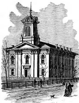
CLARION COUNTY COURT HOUSE. (From a Photograph by A. Bonnet.)
